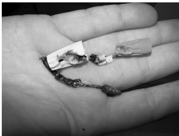
Figure 2.3: Burnt offering: Common software failures can be harder to predict and, when they occur, much harder to identify and trace than common hardware failures. (Photo courtesy of Jeffrey M. Sieracki)
