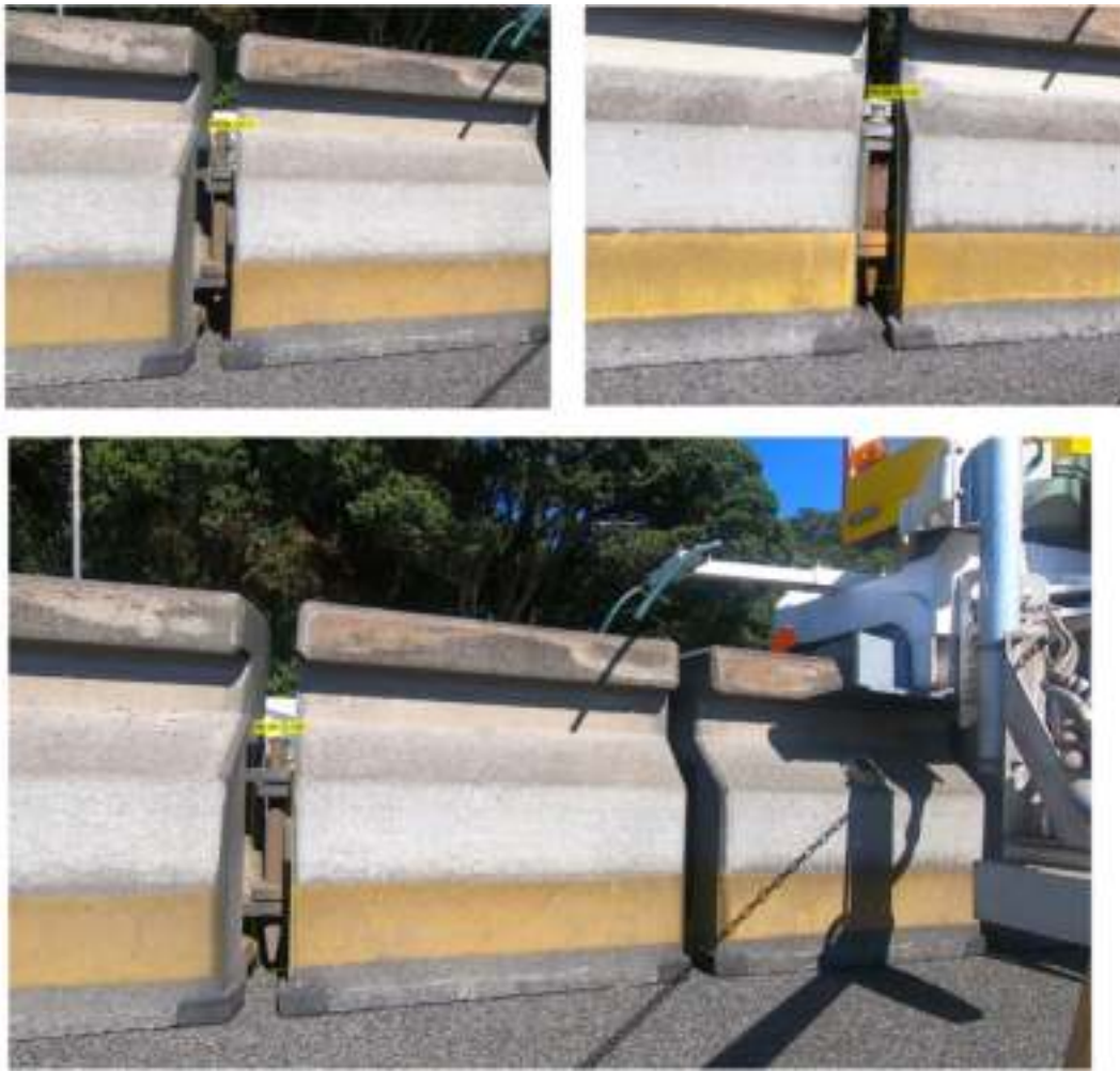
Figure 16. The selected pin ROI video frames showing generated overlays with bounding boxes.
